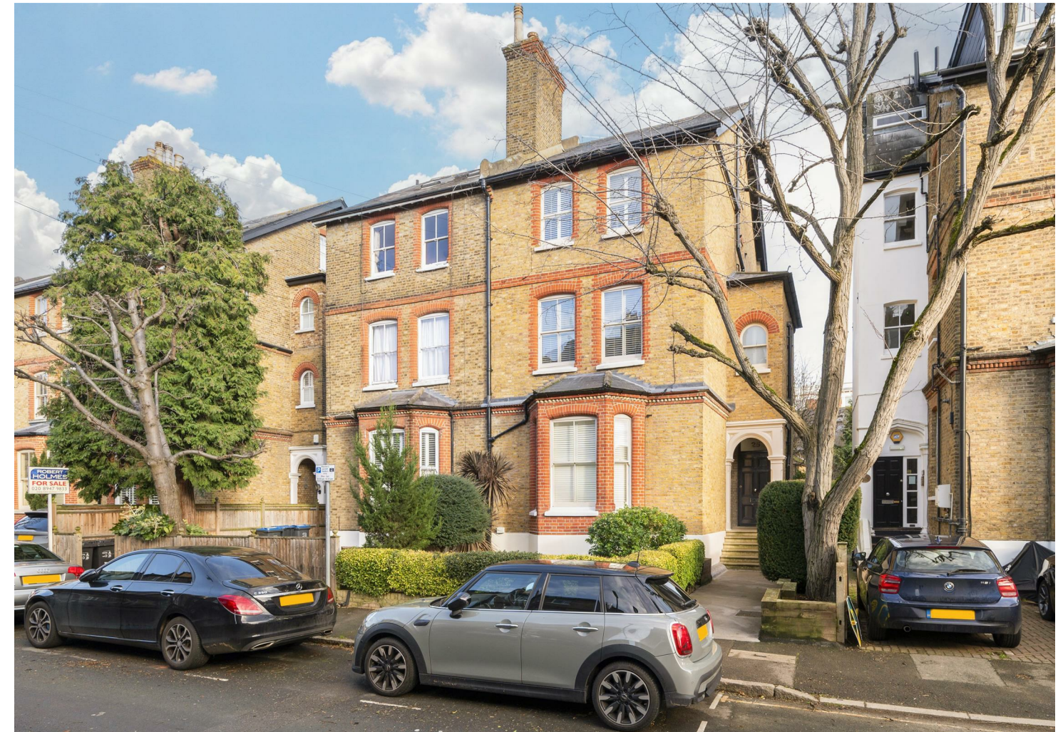
First Floor Flat, 25 Homefield Road, , SW19 4QF
